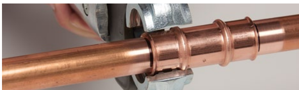
1. Insert the tube in the fitting
