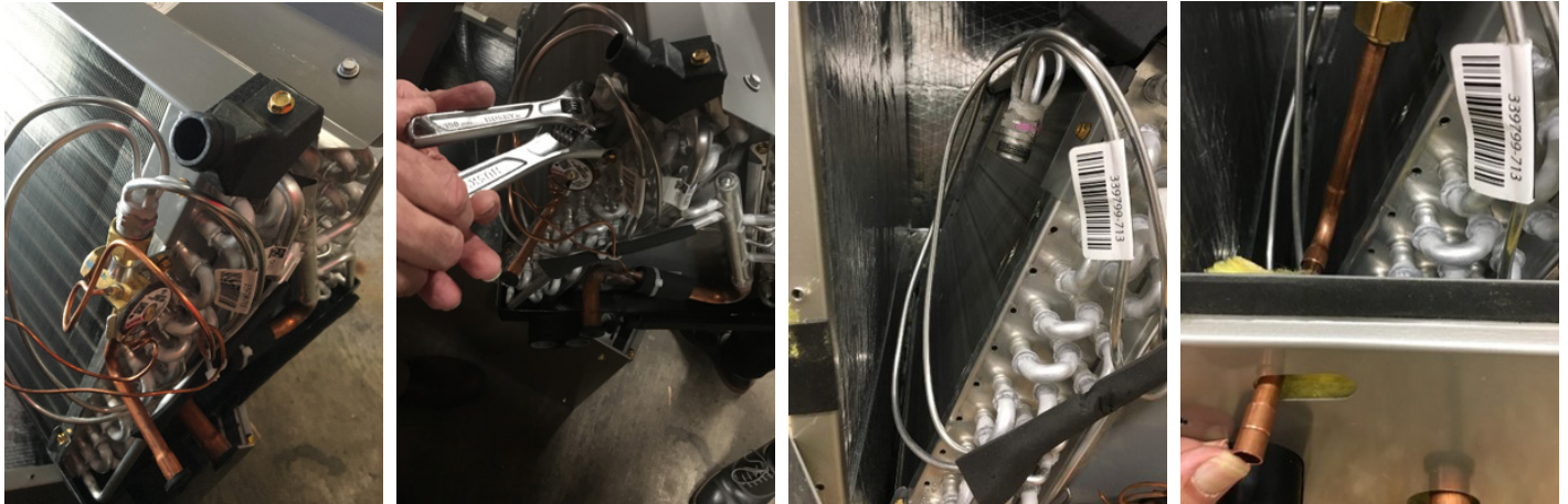
Fig. 14 — Piping Adapter Replacement
