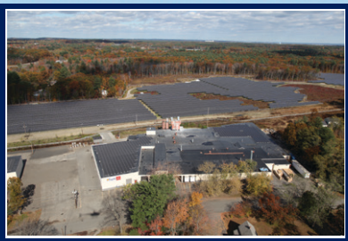
Vaughn Headquarters and Adjacent 6MW Solar Array
