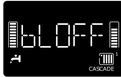
Figure 11 - Master Homescreen 3 - Boiler Off
