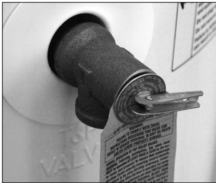
Figure 32: Temperature and Pressure Relief Valve
