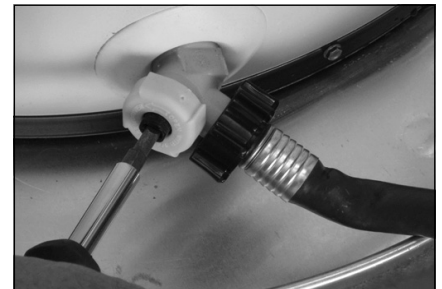
Figure 12: Draining the old water heater.
