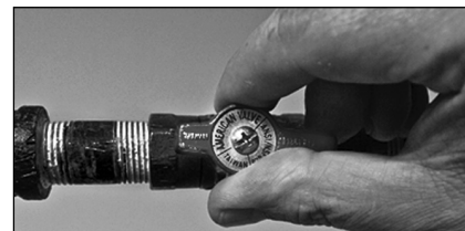
Figure 56: Gas valve in “on” position.
