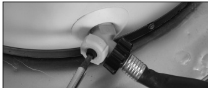
Figure 47: Draining the water heater.
