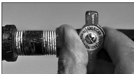
Figure 52: Gas valve in “off” position.
