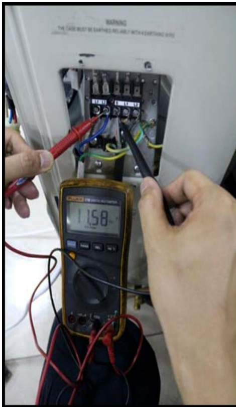
Fig. 32 – Test the DC Voltage
