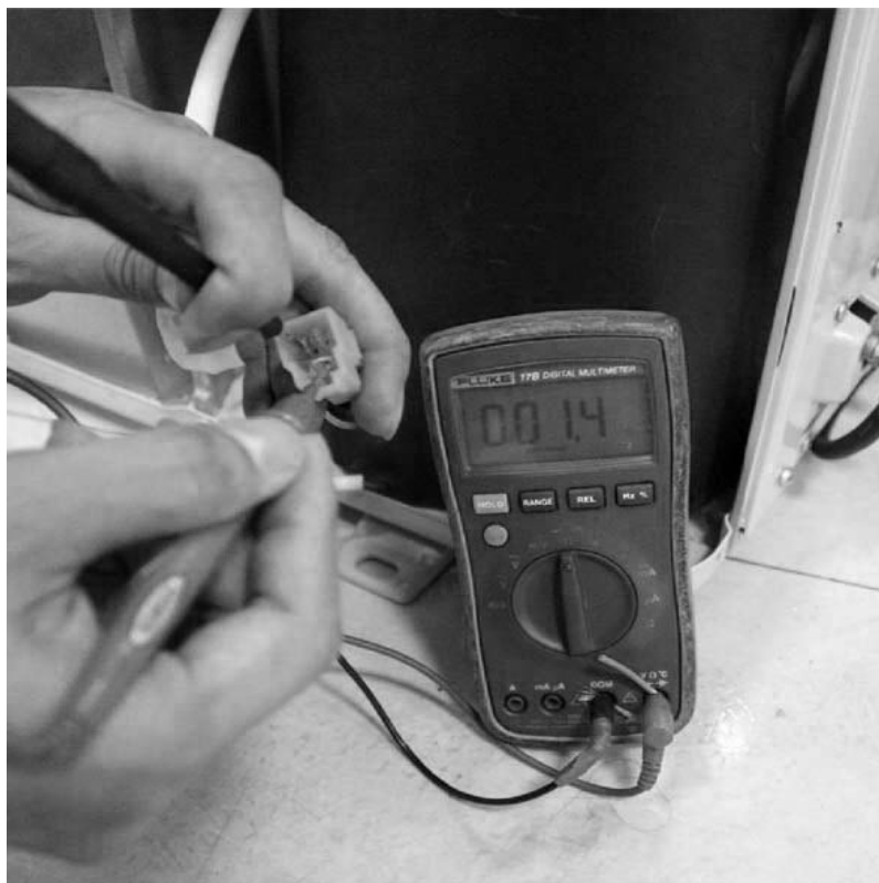
Fig. 45 – Compressor Checking
