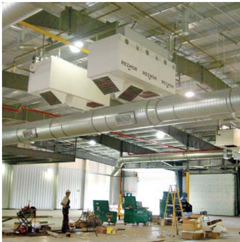
Model LDAP is arranged for vertical (downflow) air delivery. As George Reznor once said, “We live on the floor, not on the ceiling.”
